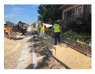
The new railroad crossing gates and lights have been installed and the conduit for the new street lights is being installed.
