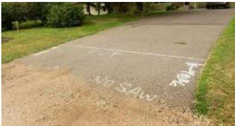
As storm sewer work wraps up, excavation of the street will commence at an approximate pace of 300 to 400 feet per day being dug down approximately 2 feet. Gravel will be backfilled at the end of each driveway so that entry and exit remains possible at the beginning and end of each day.
