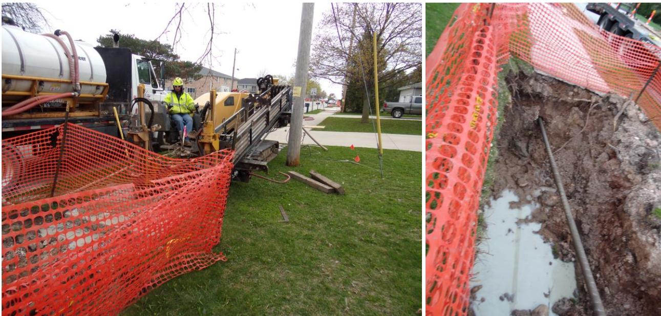
After the boring is complete, the machine pulls the new pipe through with the help of the rest of the WE Energies crew.
