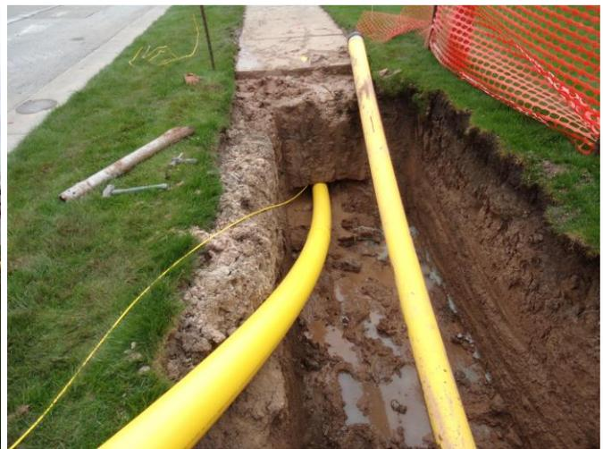
Once the pipeline is in place, work begins on service lines that run from the street to homes. This work requires We Energies to temporarily shut off natural gas service. They will contact affected residents to schedule this work, and will leave a door hanger as a reminder the day before.
