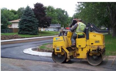
New asphalt is VERY HOT (**approximately 300°F**) when placed. Parents should keep children and pets a safe distance away from the new pavement until it cools.
