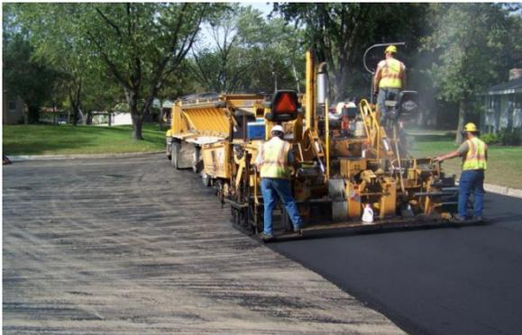
The last step in placement of your new street is laying the final lift of asphalt. Once again, you will not be able to drive on the road until they have finished rolling the newly paved road. We once again ask that you take extreme care not to make sharp turns on the new asphalt pavement.
